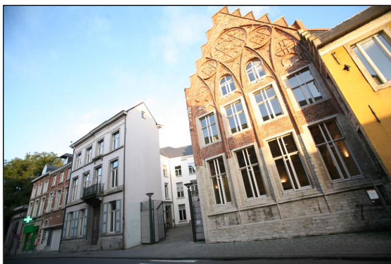
Faculty of Economics and Business - Restored historical building Naamsestraat 69, Leuven
